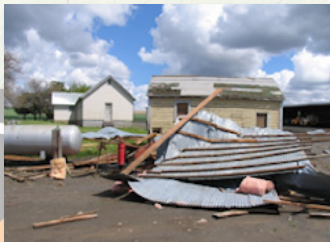
Tornado damage southeast of Adams OR, May 2009
