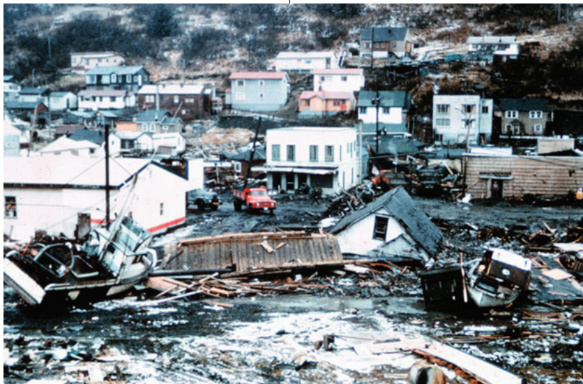
Tsunami damage at Kodiak, AK, after the 1964 Great Alaska Earthquake and Tsunamis.
