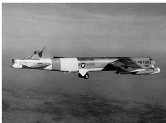
Figure 1: USAF B-52H Stratofortress flight that encountered mountain wave turbulence and lost its vertical tail, Jan. 10, 1964. Photo courtesy of White Eagle Aerospace History Blog.
