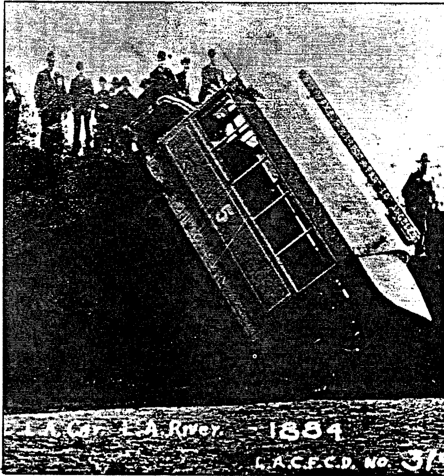
Figure 21. Flood waters of the Los Angeles River in 1884 left horse car No. 5 in a precarious position. Photo is courtesy of Los Angeles County Flood Control District.
