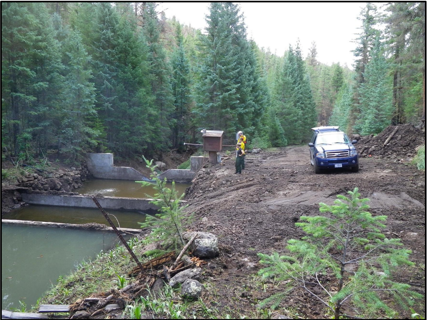
Figure 67. South Fork Thomas Creek Looking Downstream at Weir (photo provided by USFS). From High Water Marks July 11 Flow was 308 cfs +/- 20% at Weir (overtopped rectangular section by 0.67 ft).
