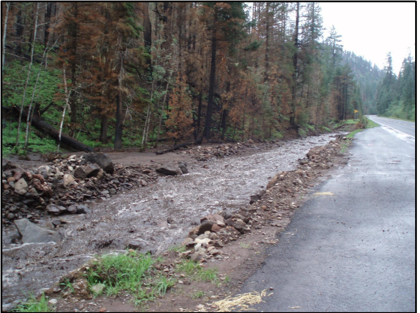
Figure 77. Looking upstream (photo provided by AZDOT, this picture was not taken on the day of storm): Cross Section #1; Channel at far end of pullout estimated as 18 feet wide at base, trapezoid shape with 30 feet wide at top, flow 6 feet deep (estimated from right bank highwater marks), wetted perimeter of 35 feet, and n value of 0.066 prior to cleaning. Slope is estimated as 0.0395 from topographic map. Estimated flow = 1,655 cfs. Mean velocity = 11.5 ft/sec.
