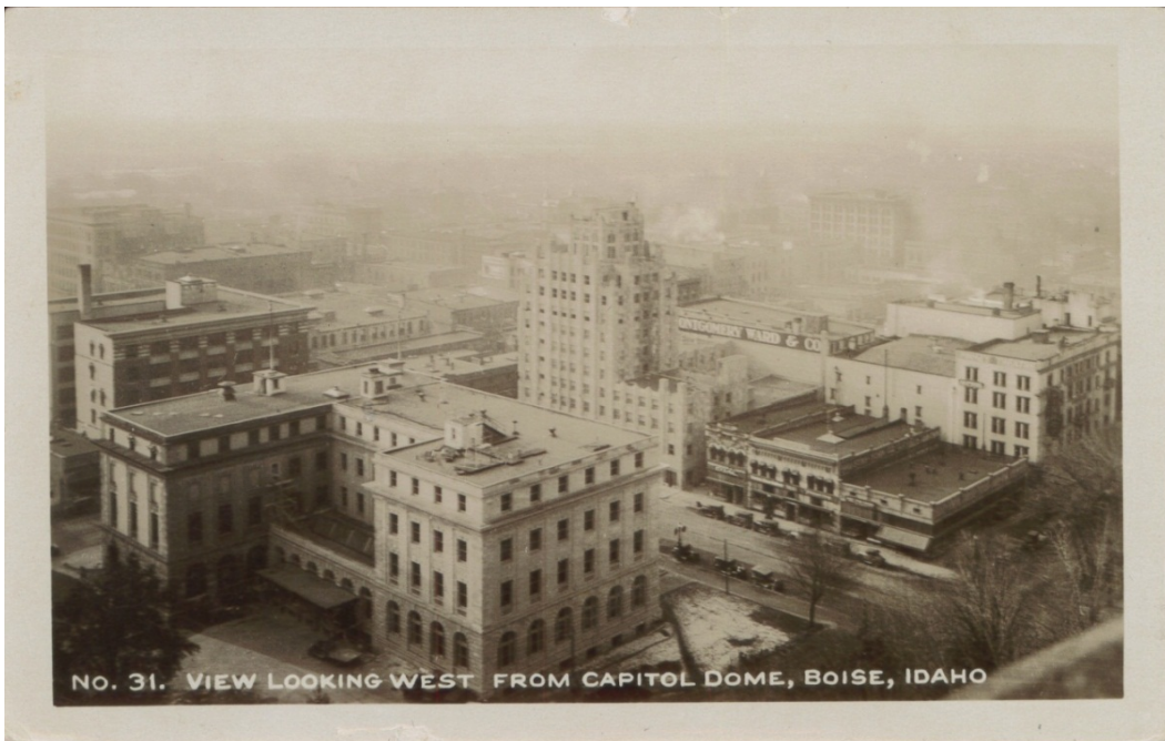
Figure 21. U.S. Federal Building with upper air observation deck and cotton region shelter on roof. Date of Photo: Circa 1930. Source: National Weather Service Boise, Idaho Archives.
