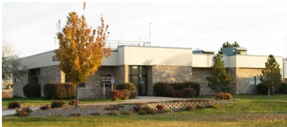
Figure 44. National Weather Service Office in Boise, Idaho looking north-northeast. Date of Photo: 2008. Source: National Weather Service Boise, Idaho Archives.
