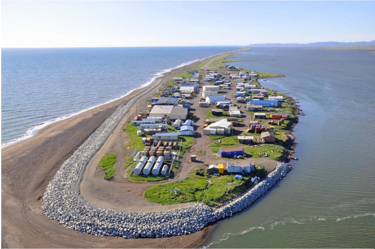
The picture above shows the community of Kivalina, located on the coast of northwest Alaska. The shoreline armoring in the foreground is evidence of extensive efforts to reduce erosion and protect the community from further impacts. Credit: ShoreZone Survey
