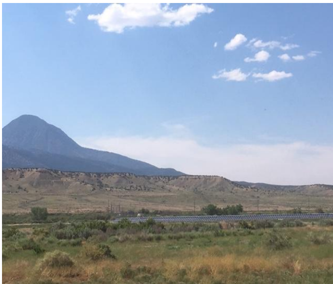
Towaoc Community Solar power plant—over 3,600 PV panels, creatively net-metered; Ute Peak in background.
