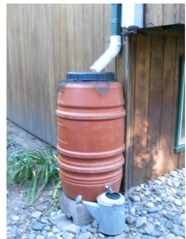
Rain harvesting barrel can be used for collecting rainfall from a rooftop. Photo by Susan Wotkyns.
